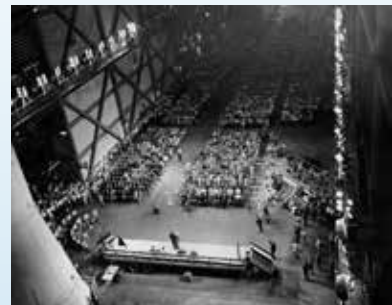
Most of the Launch Support Team gathers in the aisles of the VAB to hear the astronauts thank us for a job well done
